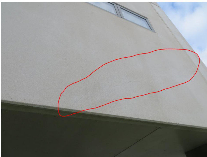
Figur 11: Revne i betonelement
